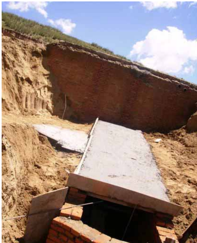
Building the cistern.
