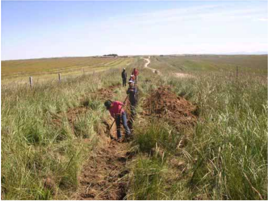
Locals dig the ditch for the pipe.
