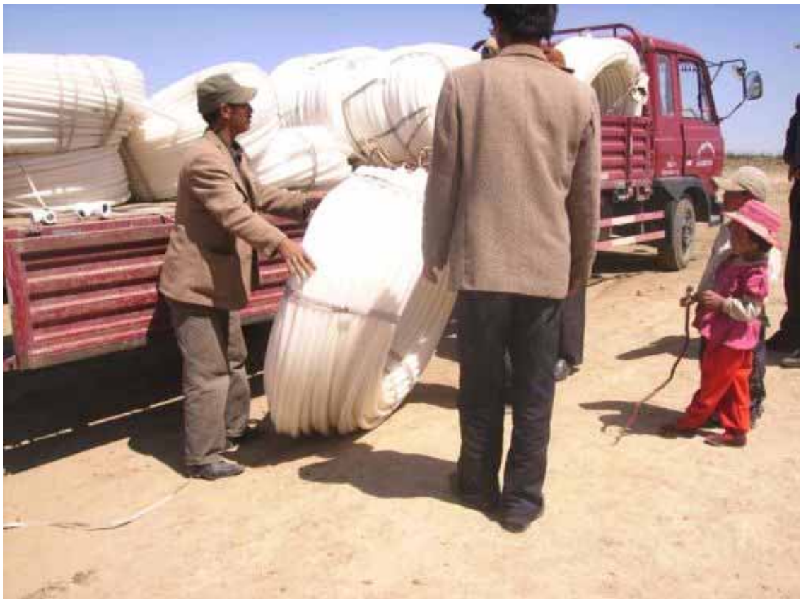
The pipes arrive in Bon skor Village.
