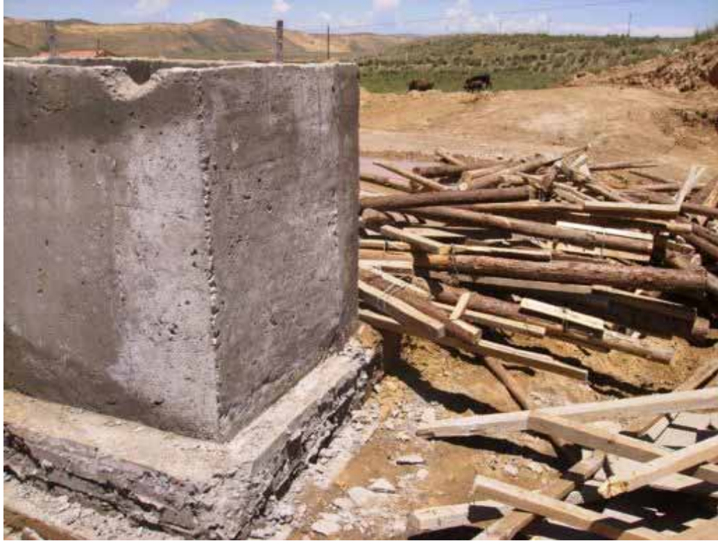
The cistern top--the main body of the cistern is underneath.
