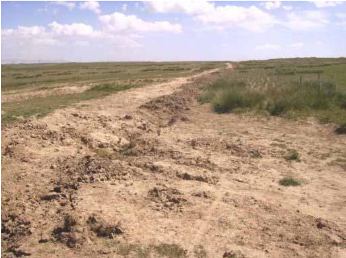
Ditches are filled in.
