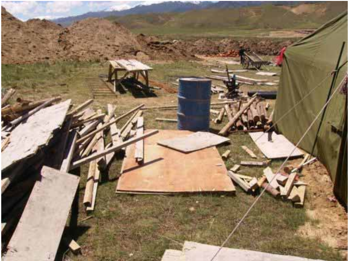
Local workers prepare to build the cistern.
