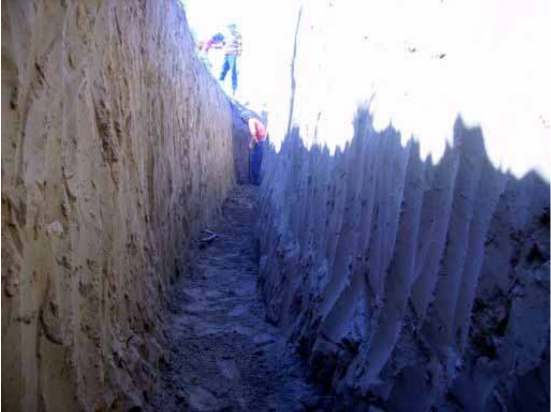
Ditch digging is complete.
