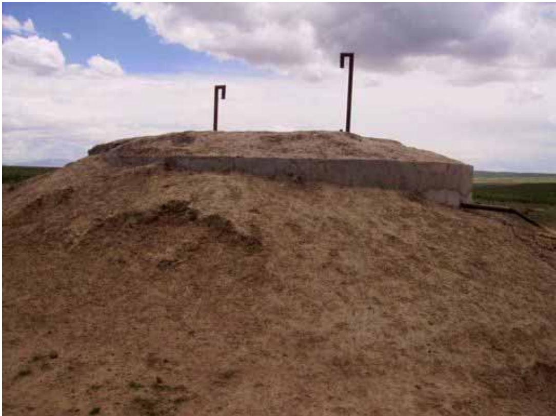
Completed cistern--pipes allow for air intake.
