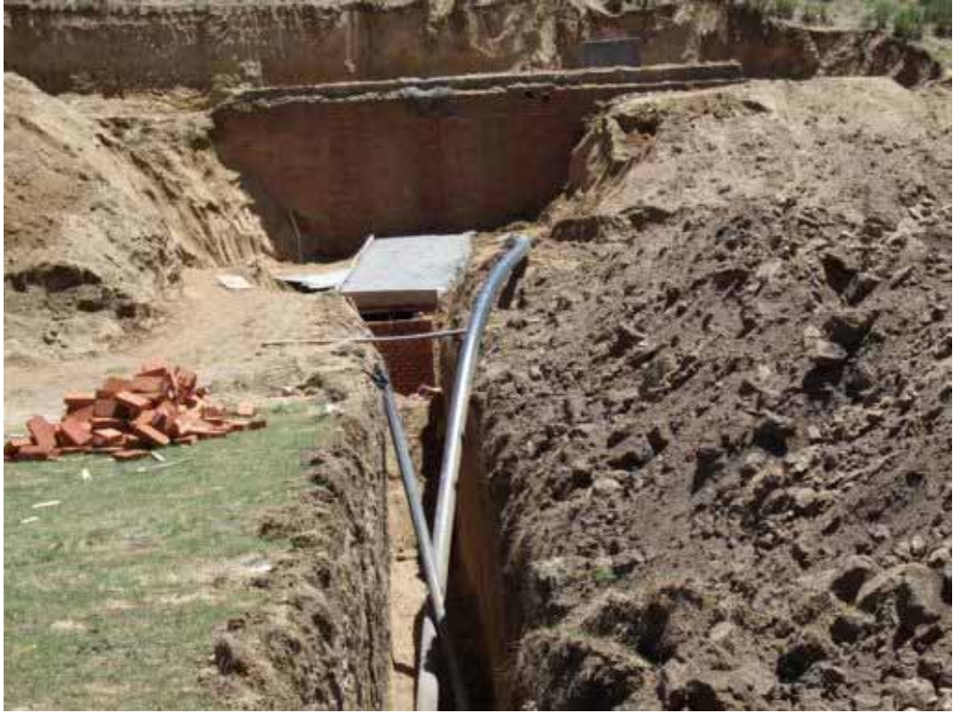
Building the cistern.
