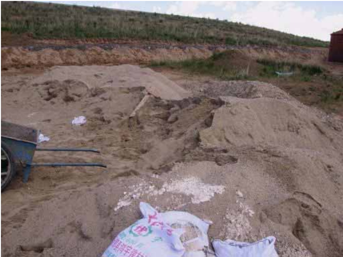
Sand for cistern construction.
