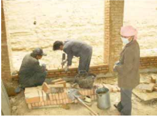
Workers build clinic foundation.
